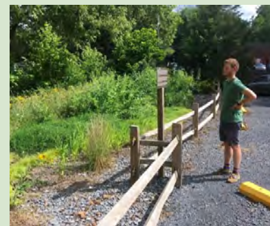
Split-rail fence creating a boundary between the parking lot and a rain garden/riparian buffer.
